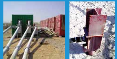
Biofilter facilities for aeration of the landfill areas and connection to lance cap
