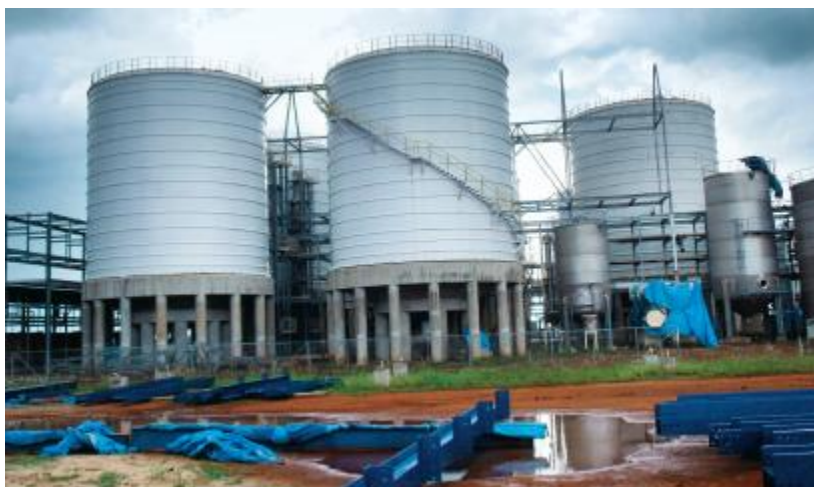
The TPK plant in Thailand where a 30-year old coal boiler is currently being converted to run on biomass. On the foreground is the foundation where the boiler will be erected (photo credit: DP CleanTech)
